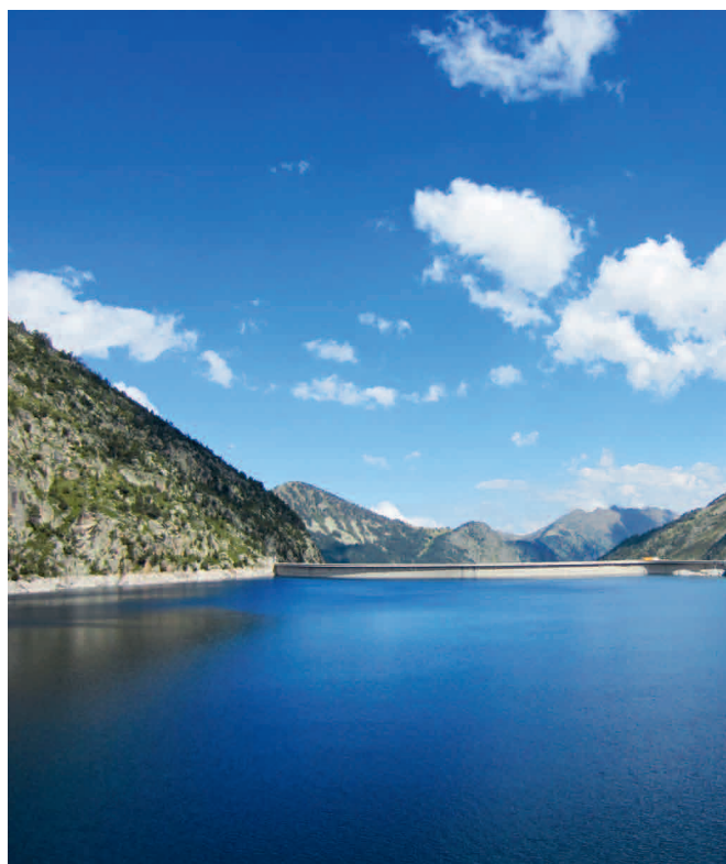
Reservoir in France 2012
