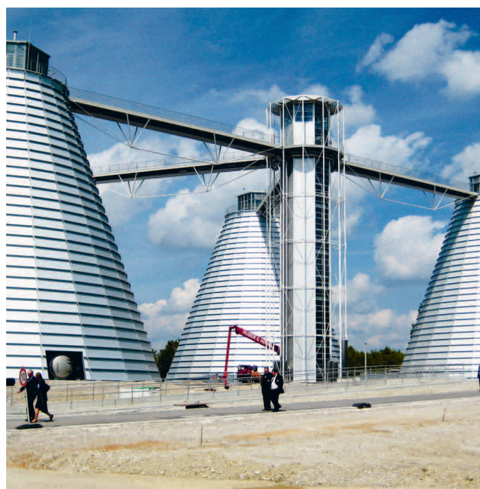
Wastewater treatment plant Munich, Germany 2010
