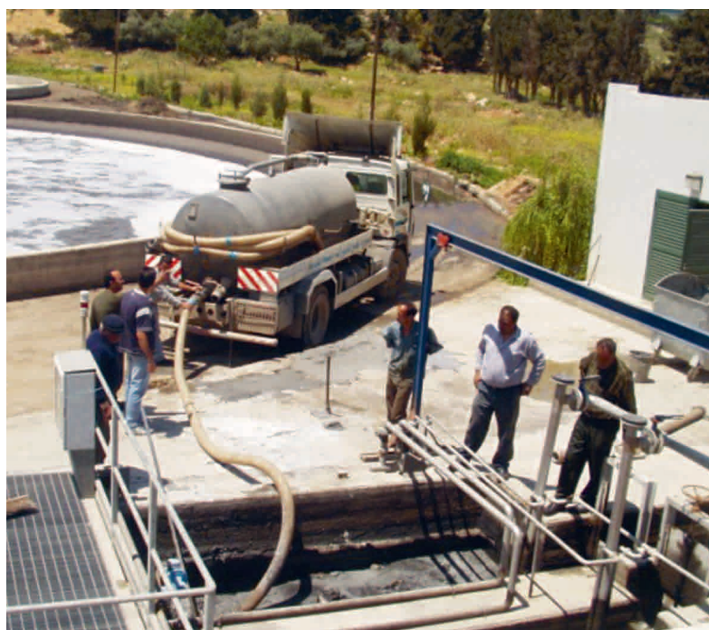
Wastewater treatment plant in Palestine, Ramallah 2005
